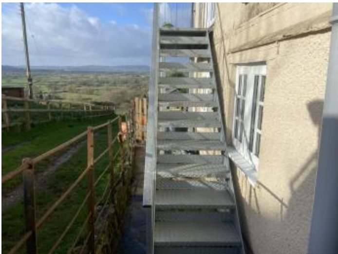
Metal stairs towards entrance of Strongate View Apartment
